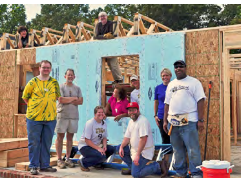
ZSR faculty and staff volunteer at the Wake Forest Habitat for Humanity house.
